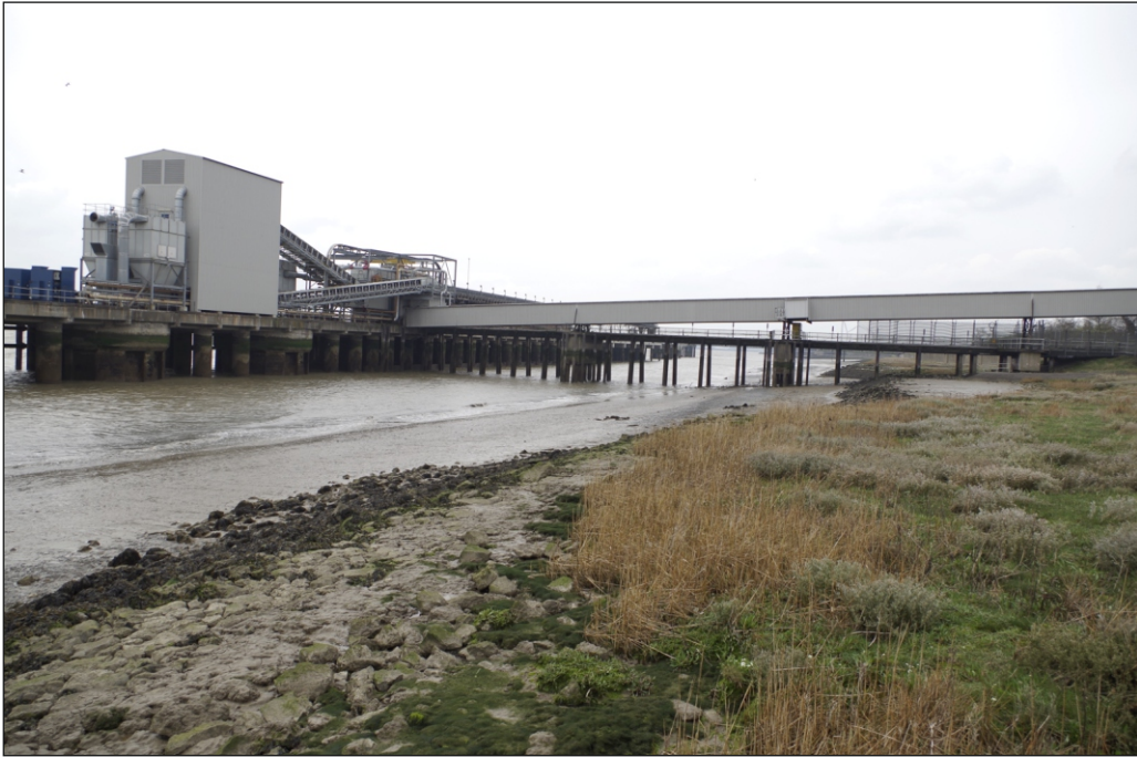
Plate 3: View from foreshore of Tilbury coaling jetty covered conveyor, facing SW
