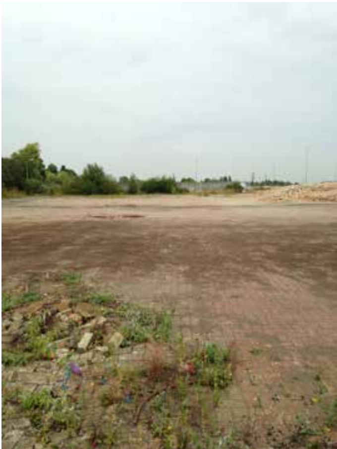
Plate 20: Paved former yard surface
