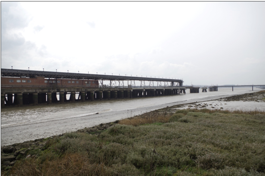
Plate 2: View from foreshore of Tilbury coaling jetty, facing SW
