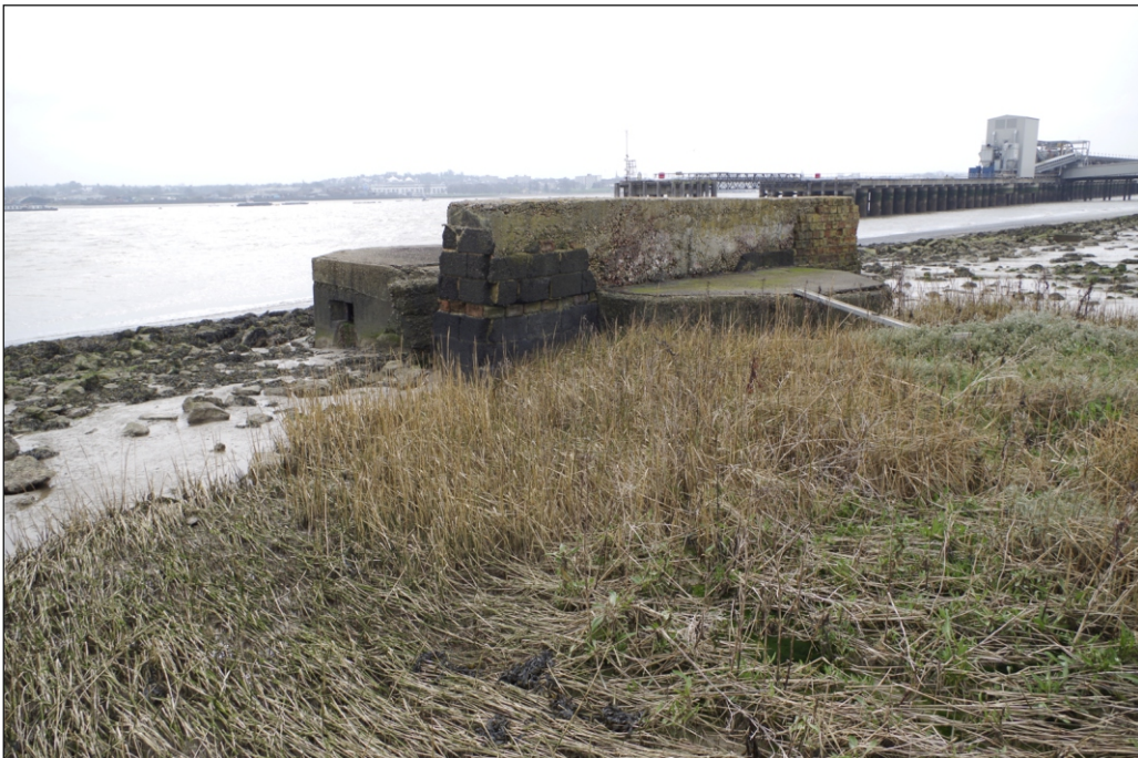
Plate 4: Pillbox WA 1001 in inter-tidal mud facing SW
