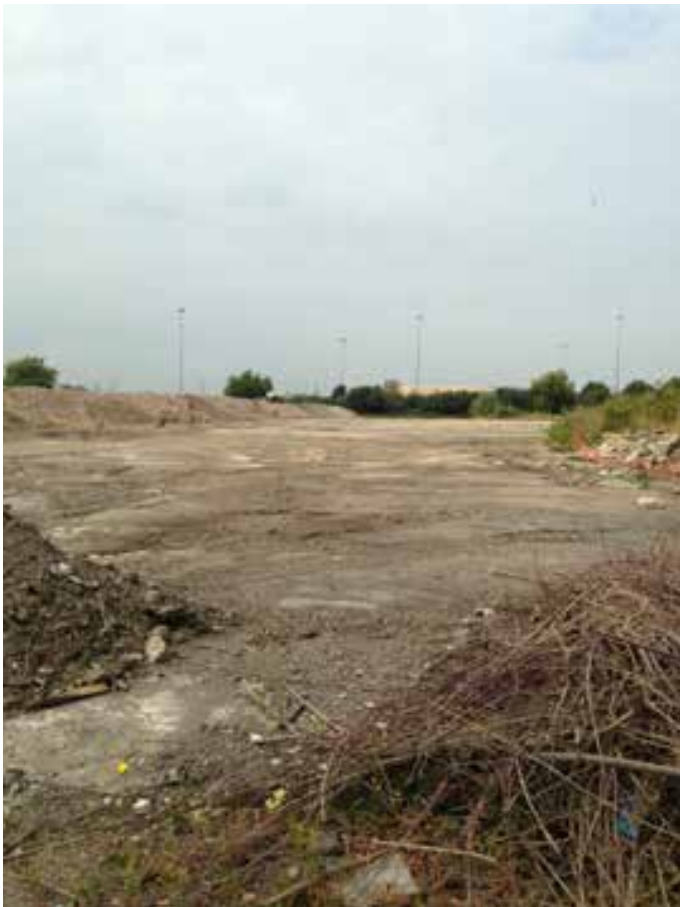
Plate 14: West facing photograph showing site clearance
