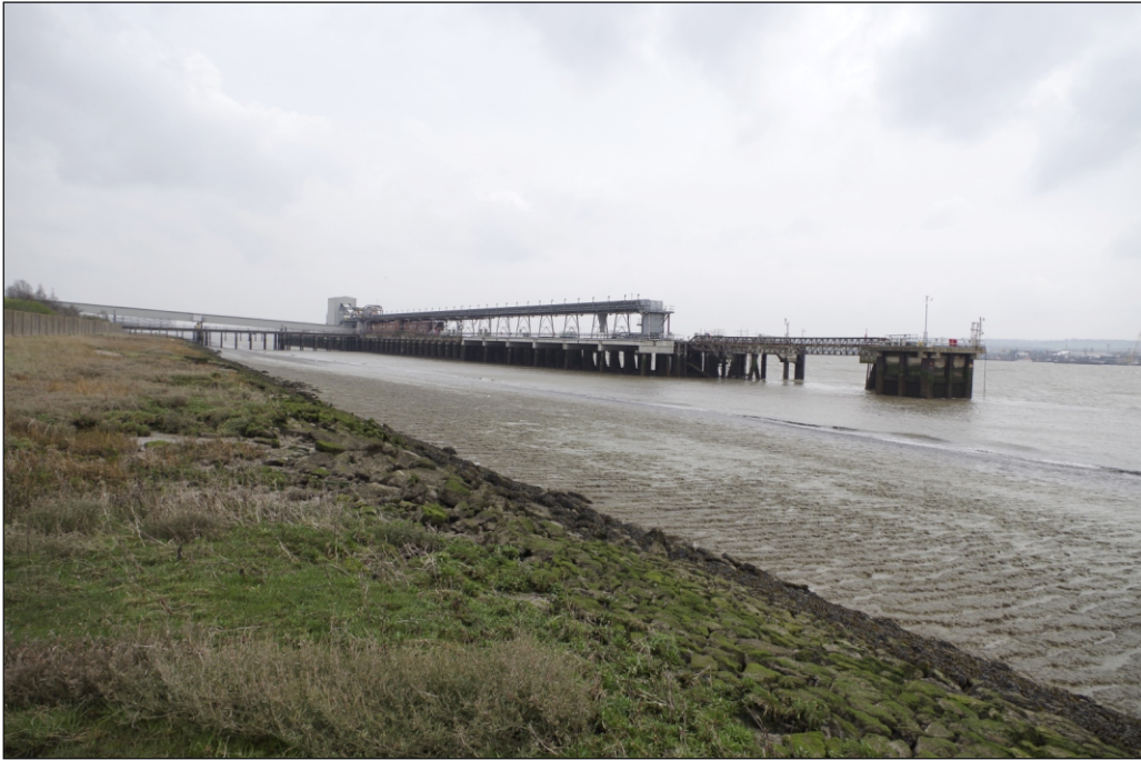
Plate 1: View from foreshore of Tilbury coaling jetty, facing SE
