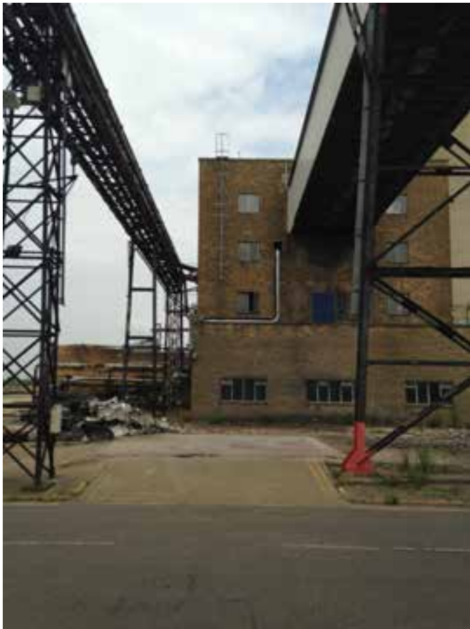
Plate 7: South facing photograph of extant former Tilbury A building and conveyor belt
