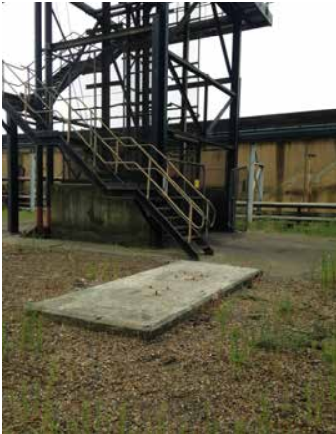
Plate 5: West facing photograph of rectilinear building in the eastern boundary of the study site with steps accessing the conveyor belt in the foreground
