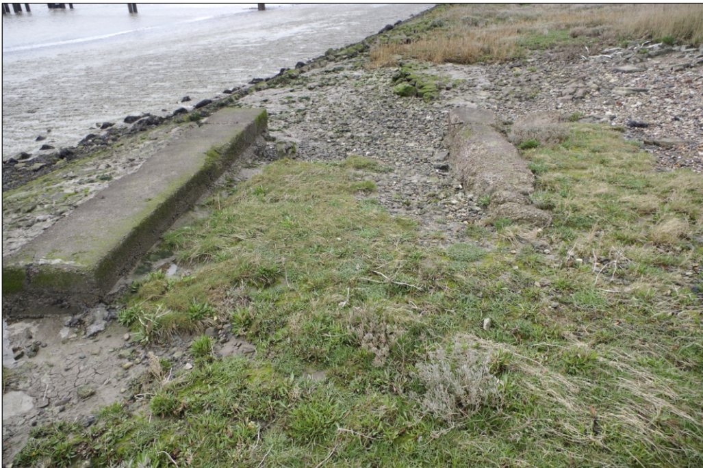
Plate 8: Undated concrete feature on foreshore, facing SW (WA 1020)
