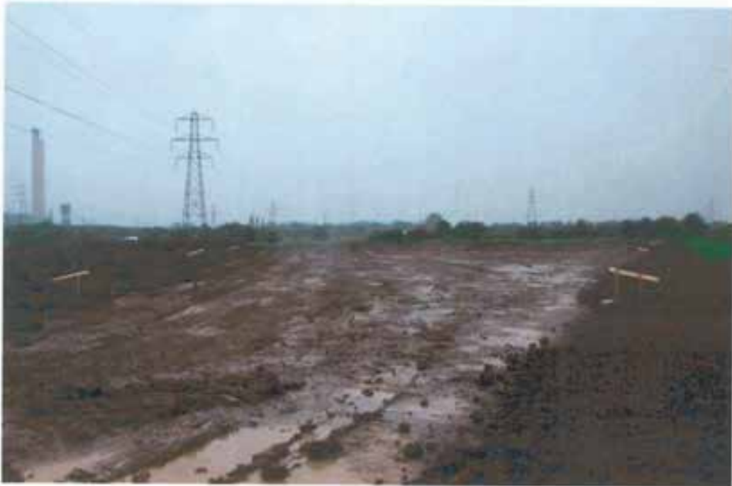
Plate 2. Bund area stripped but obscured by plant tracks.
