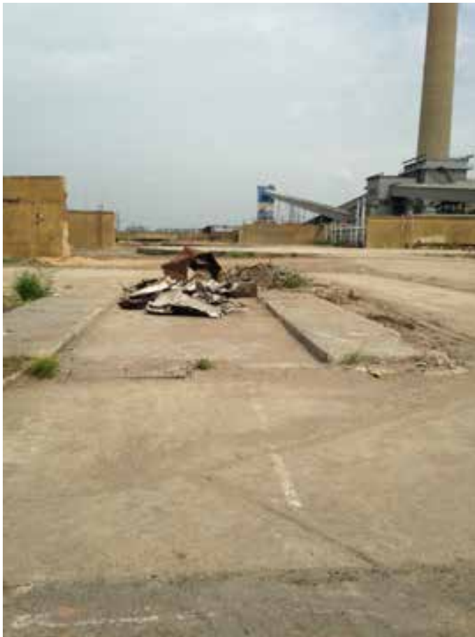
Plate 15: North facing photograph looking towards the former circular tanks (concrete slab still in situ) in the east of the site
