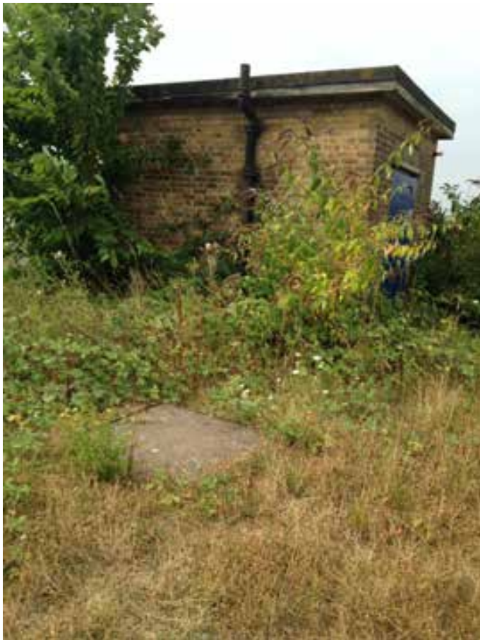
Plate 2: Small single storey sub-station in the east of the site
